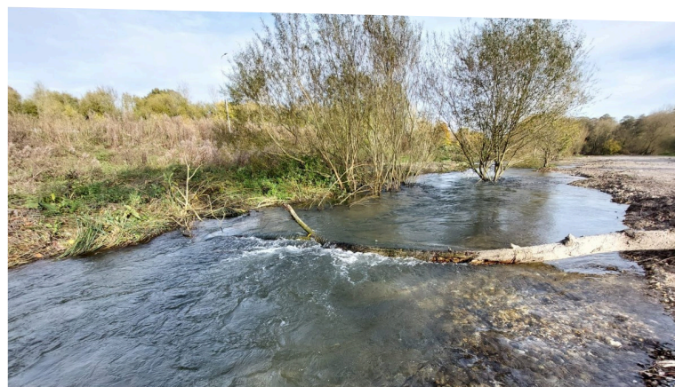
Installed habitat features
