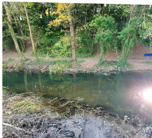
Added gravel and wood to improve flow rates and provide cover and marginal areas.
