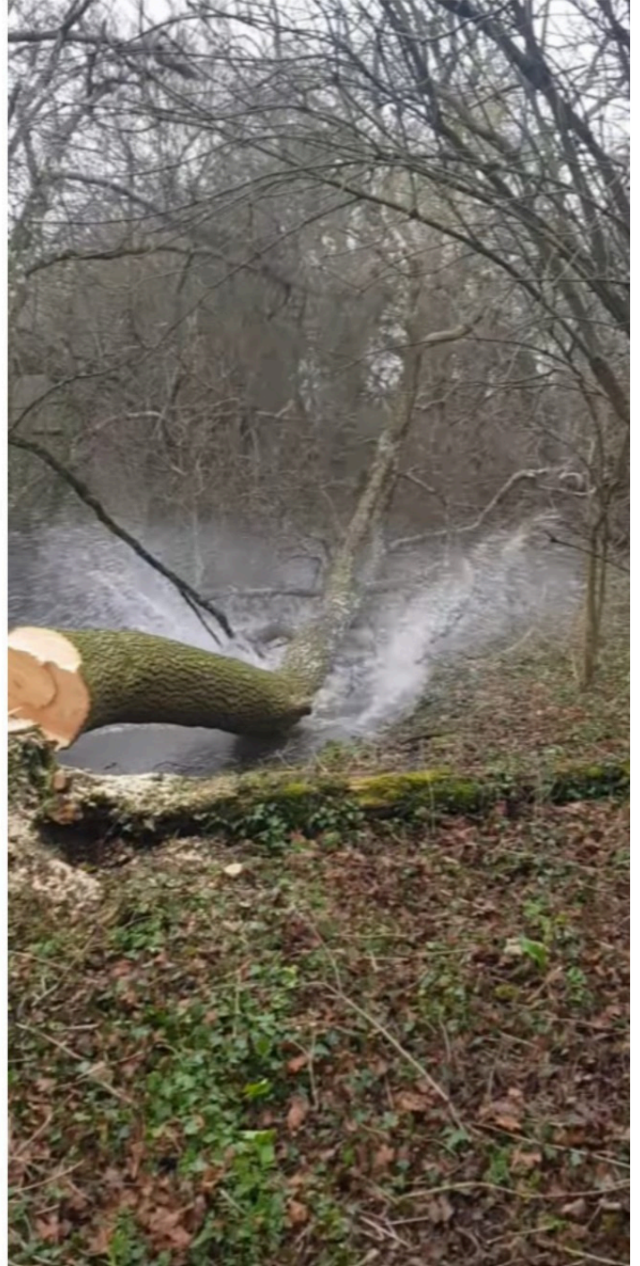
A diseased ash tree felled into a perched (realigned to the valley side) winterbourne channel. The resulting log jam will encourage flows to breach into the adjacent floodplain, reconnecting the river with the landscape and creating new wetland habitats. Nature-like interventions such as these are low cost and quick to install.
