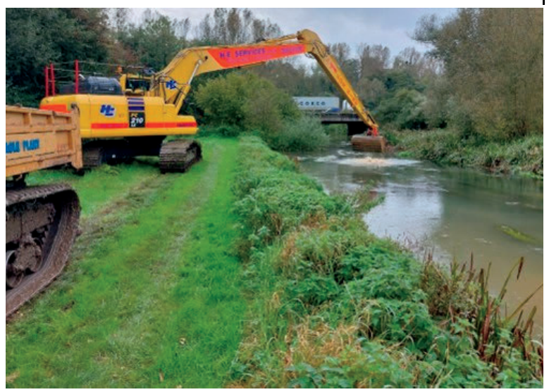
Long reach excavator installing gravel into the river channel.
